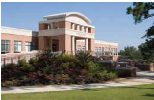
Meisler Hall - Gray metal roofing, Railings, trim
