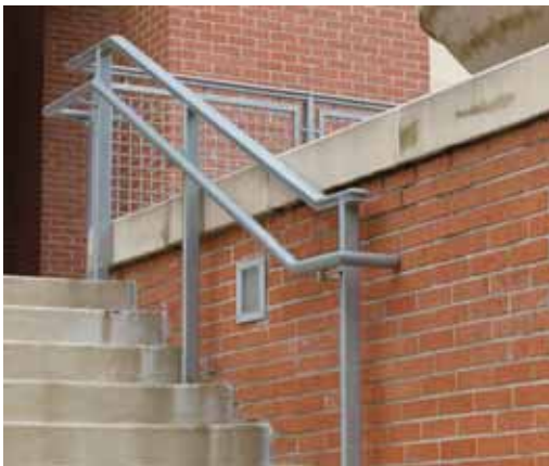
Gray Metal Railings/Trim
