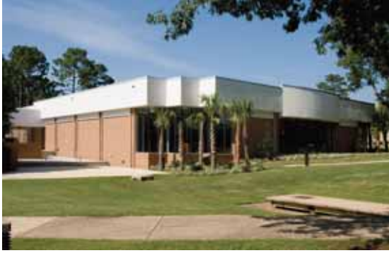
Stucco at Cornice
